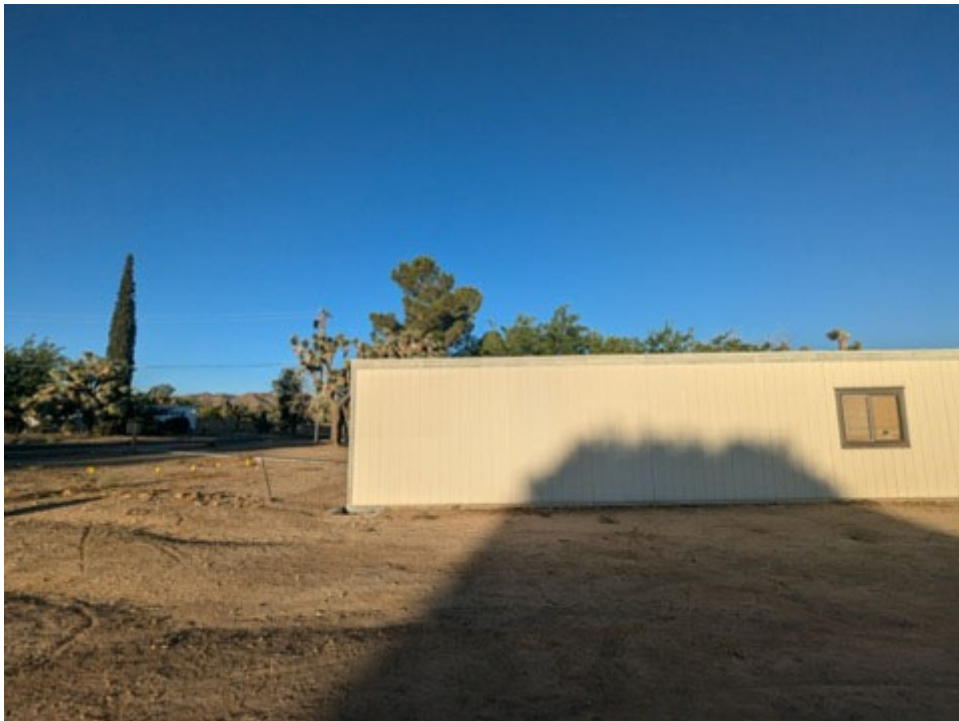
West facing view from the project site.
