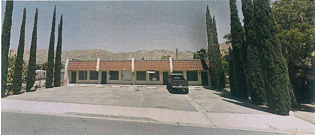
South (Front) Facade:
