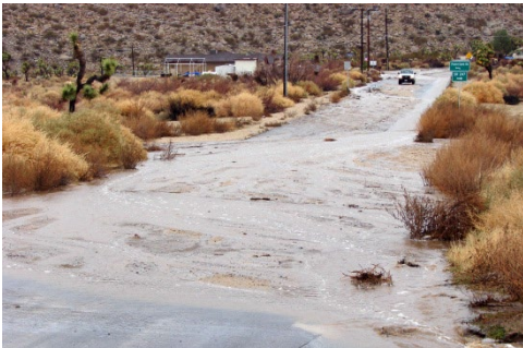
Floodwaters inundating a low-lying roadway.
