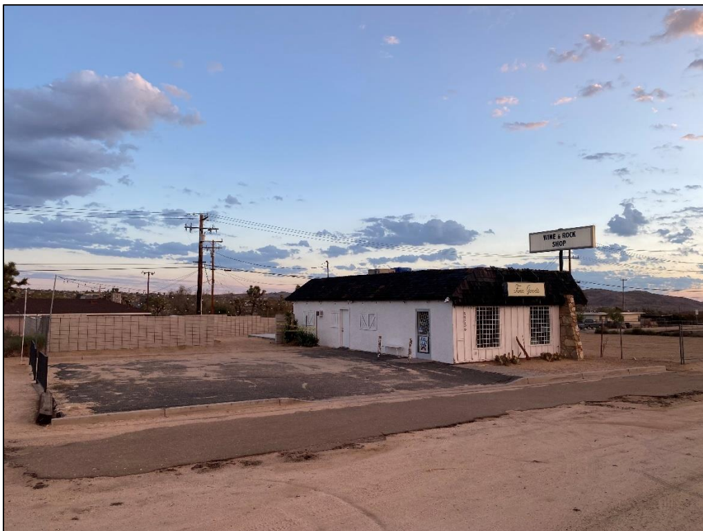
Figure 2. Southwest corner of Wine and Rock Shop, looking towards center of property.
