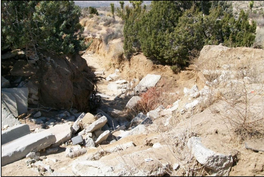
Figure 8. Overview of drainage/wash, view to west
