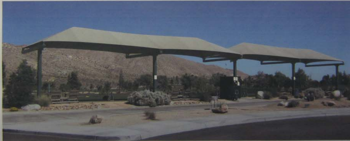
VACUUM STATION SHADE STRUCTURE
