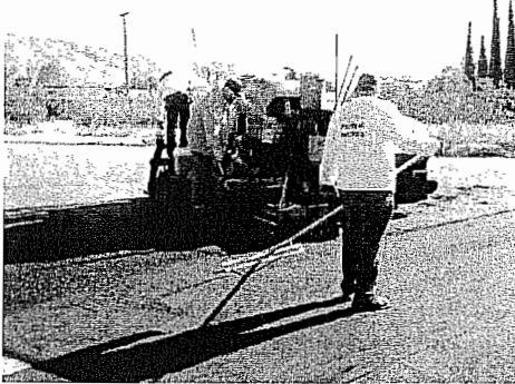
Public works staff paving a road in Town.
