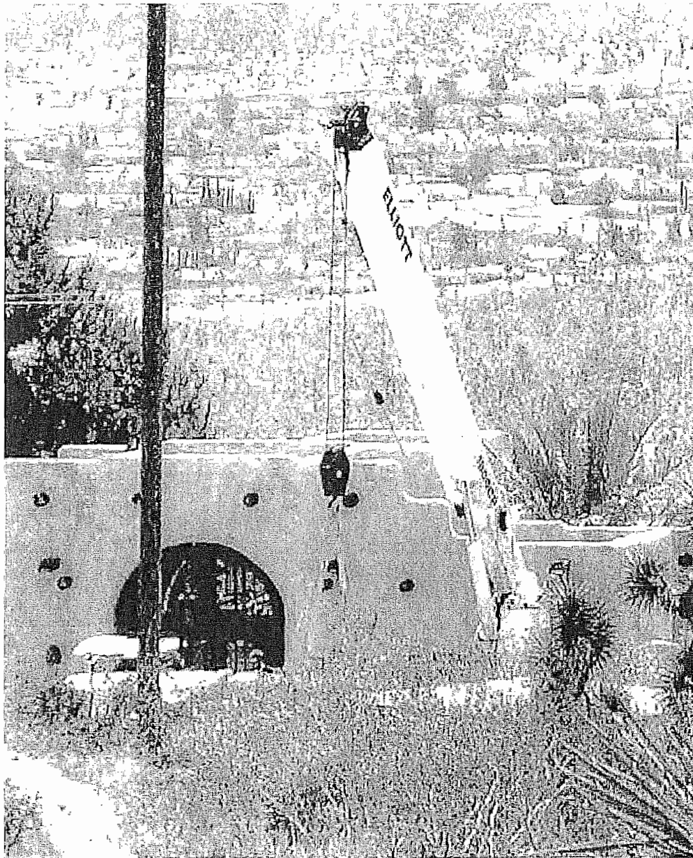
Heavy lifting crane in operation at situs of HOP 11-05.
