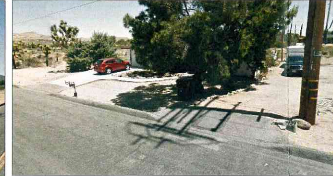
Across the street from central YVHS parking lot on Sage. Proposed sidewalk will have gaps where there is existing residential access. Budget pending existing AC dikes and driveways may be demoed and rebuilt along with sidewalks for a continuous concrete pedestrian path.
