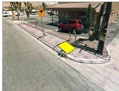
NEC of Sage Avenue at Jamie Ann Lane. Full width of sidewalk to be constructed with ramps at Jamie Ann. Some relocation of signage may be required from the alleyway to Yucca Trail with utility protection.
