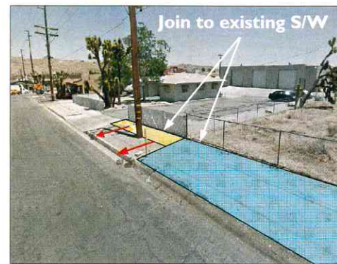
SWC of shopping center at back warehouse parking lot. Proposed sidewalk/C&G shall connect to the existing sidewalk at full 60" width.
