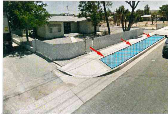
SEC of Sage Avenue at Jamie Ann Lane. Full width of sidewalk to be constructed/completed from existing pedestrian walkway to curb.
