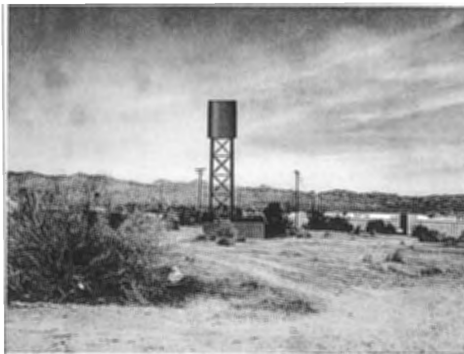
PROPOSED INSTALLATION OF '65 STEALTH WATER TANK WITH ANTENNA ARRAY, ALONG WITH INSTALLATION OF EQUIPMENT COMPOUND SCREENED BY A 8' BRICK WALL.
