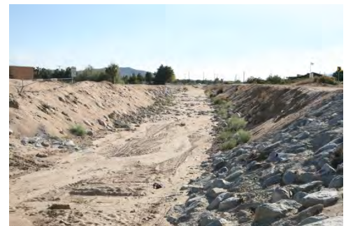
Unlined drainage channels are part of the Town's stormwater runoff management system and provide opportunities for new trail linkages.
