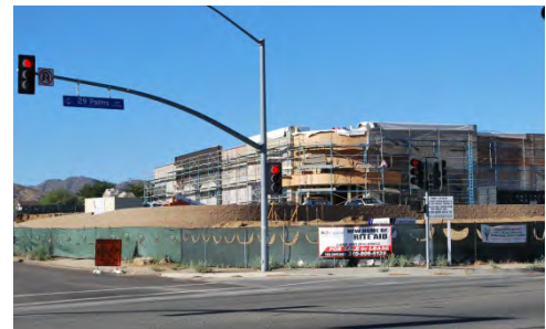
Construction is an example of a temporary source of noise.
