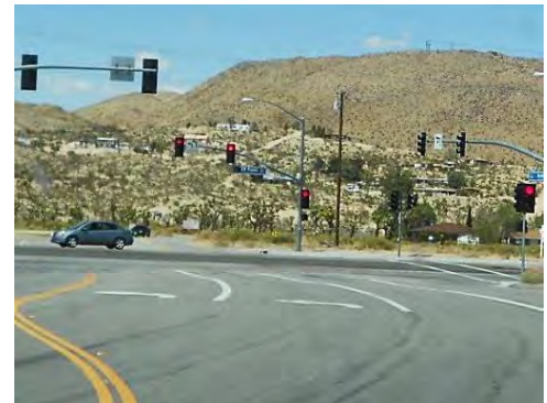
Avalon Avenue is a collector roadway with a level of service of C or better north of the intersection with SR-62.
