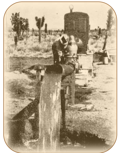
First Yucca Valley Village County Water District Well Source: History of the Morongo Basin
