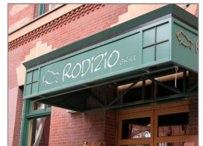
Awnings and canopies also provide protection for pedestrians.
