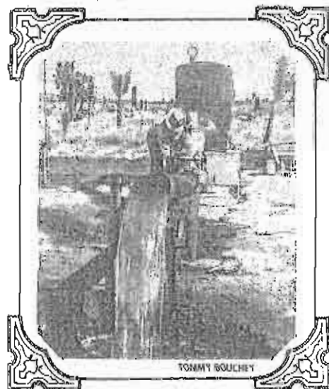
FLOWING WATER, at last. No more water hauling.
